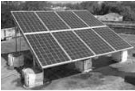
Fig.3: SPV panels installed at CNT
